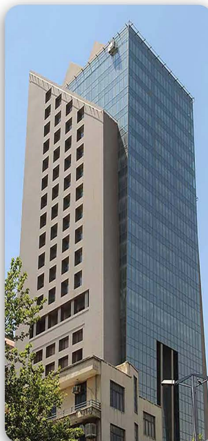
▲ Omid 2 Tower (Indoor Lighting)
