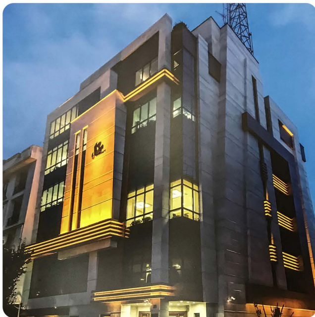
▲ Mahtab Bld (Indoor, Facade & Landscape Lighting)
